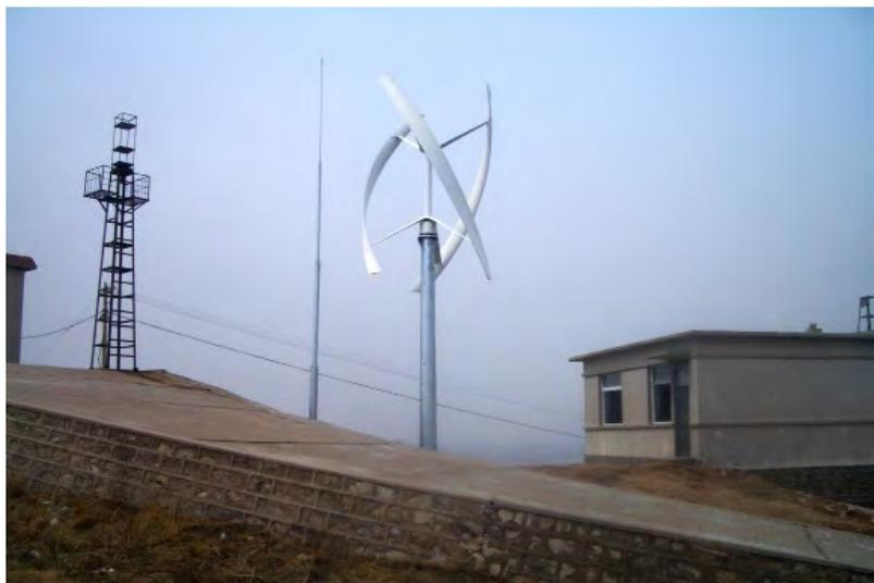
In July 2011, the Chinese Navy installed an **Urban Green Energy Fusion system** at a coastal location on mainland China to power one of their communication towers. The system consists of an off-grid **UGE-4K vertical axis wind turbine** with **2 kilowatts of solar**.
